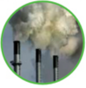
Coal Power Plant
